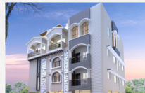
CLIENT NAME -MR.VAIDEESWARAN AREA - MALLESHPALAYA, BANGALORE CONSTRUCTED AREA - 13500 SFT
